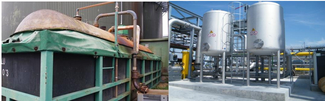
Pictures: In Situ Desulfurizer (left) and Activated Carbon Desulfurizer (right)
