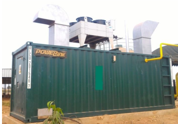
Picture: CHP in Container with all accessories
