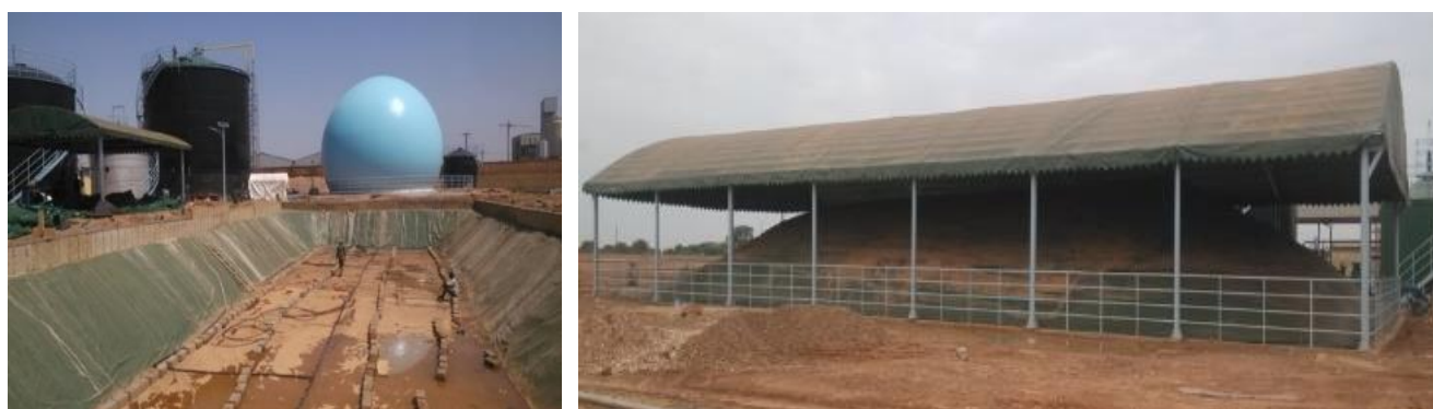
Picture: Construction phase and installed covered lagoon digester.
