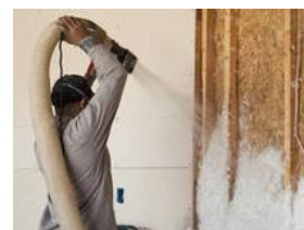
Fig. 36: Blown-in insulation
