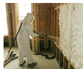
Fig. 37: Foamed in place insulation
