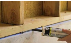
Fig. 43: Sealing foundation and framing
