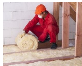
Fig. 35: Insulation through blankets
