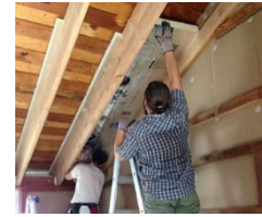
Fig. 38: Insulation using rigid boards
