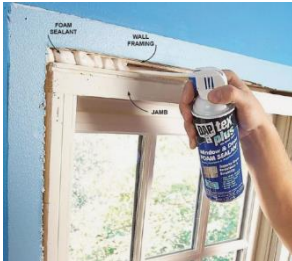
Fig. 44: Sealing wall and window gap
