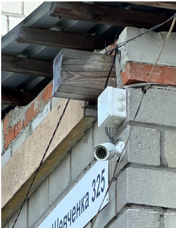
The existing video surveillance system and its connection. According to the project, preliminary dismantling and replacement. Photo
