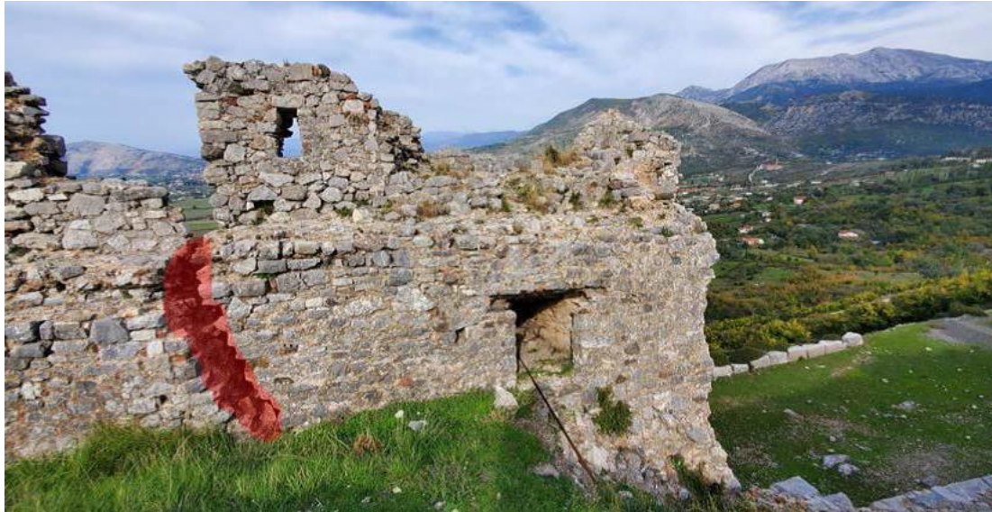
Structural Wall crack
