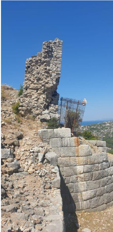
From the careful observations in the field, it is noticed that the wall has problems related to its stability since the wall has acquired a slope which causes it to be eccentric in the action of the normal force, a reason which can cause it to collapse and be destroyed.
