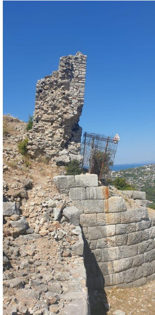
3. The increase of the soil level behind the wall over time, due to the movement of soils as a result of atmospheric agents, and not only. Since the wall in this area was the end part, it also served as a place for depositing soil. The increase in earth pressure on the wall has exceeded the bearing capacity of the wall, leading to its damage.
