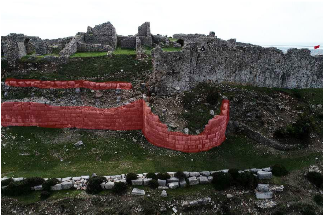
Damage to the lower part of the stone masonry
