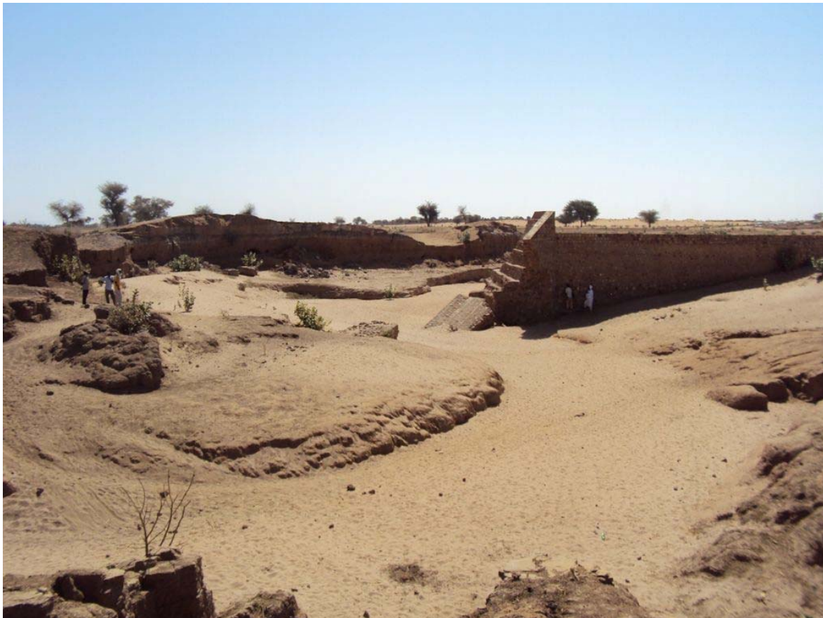
Photo 2: Breach adjacent to Secondary Spillway viewed from upstream looking downstream
