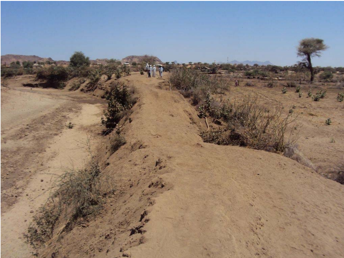
Photo 4: View "A" eroded embankment looking North
