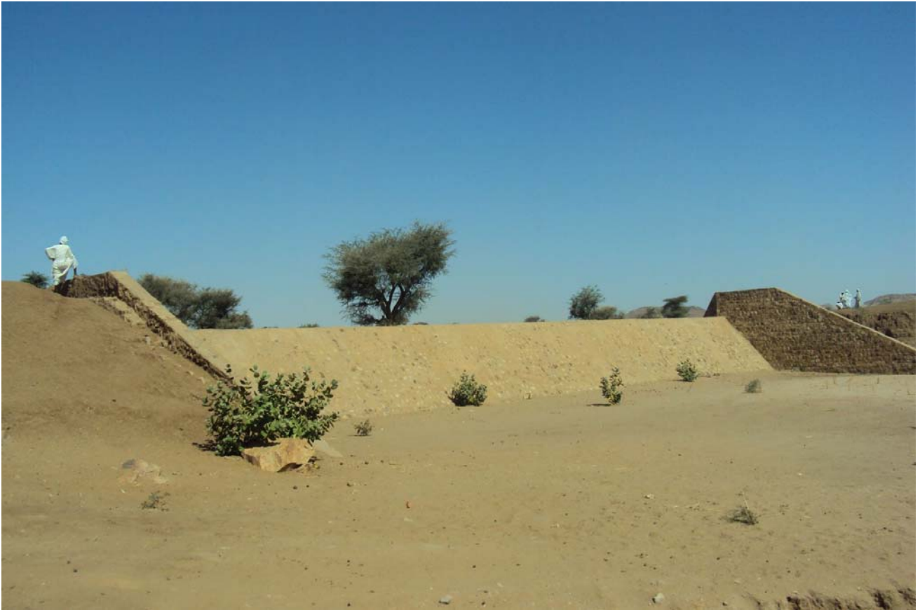
Photo 7: Secondary Spillway viewed from downstream. Breach section is at RHS of photo.
