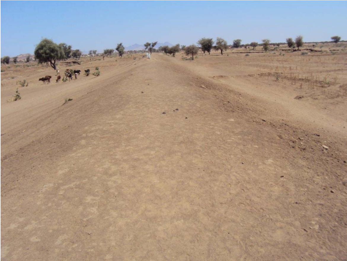
Photo 5: View “B” eroded embankment looking North
