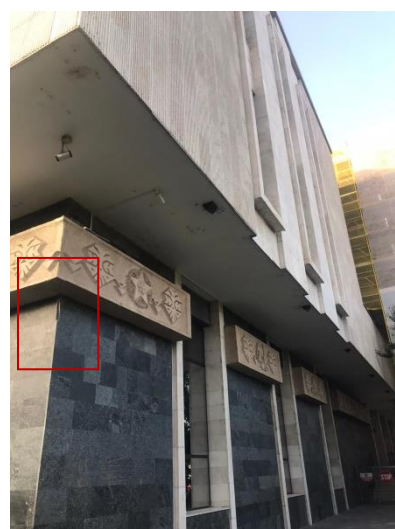
Fig. 11 Cracked tiles on facade
