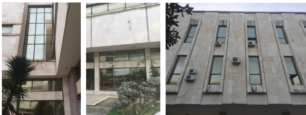
Fig. 7 Cables, installations and air conditioners on the facade
