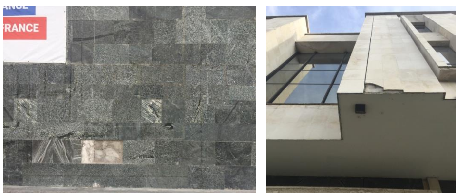
Fig.13: Damage to tiles and finishes
