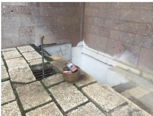
Fig. 14 Damaged floor tiles
