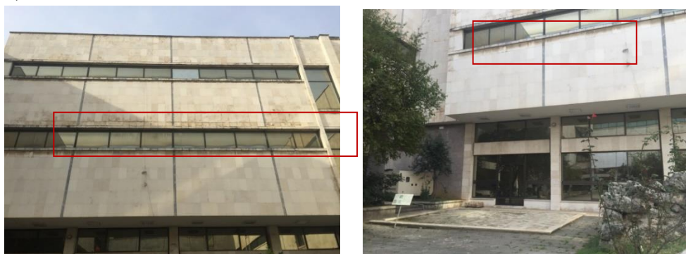
Fig. 5 Impurity on the facade by atmospheric agents
