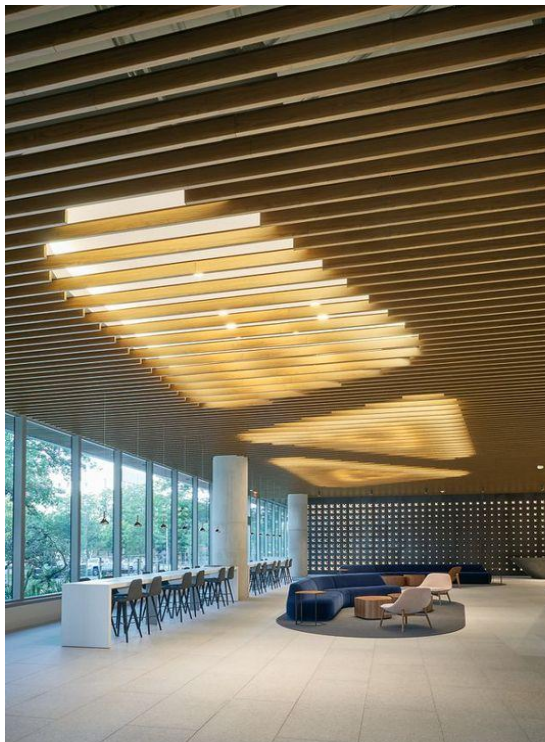
Acoustic Panelling Type 5 Baffle Ceiling - Learning Commons & Common Areas
