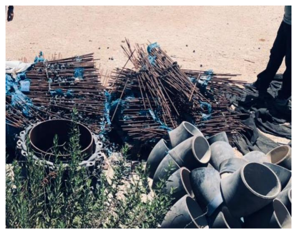
Rusted Reinforced Steel shall not be used in the project.
