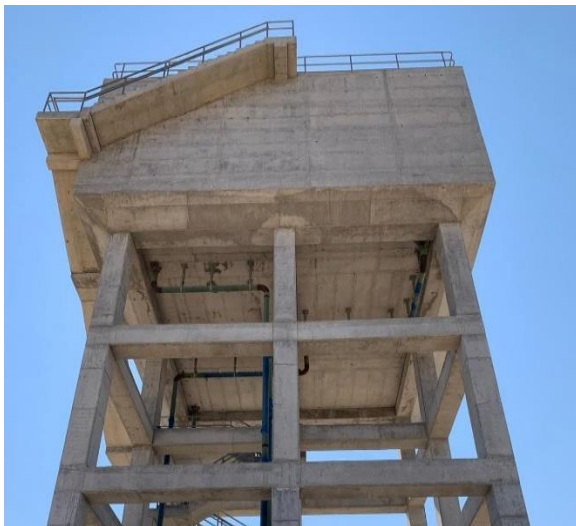
The body of the tank is not painted. The tie rods locations must be treated.
