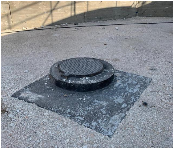
Reservoir yard level is not reached. Additional layers are required
