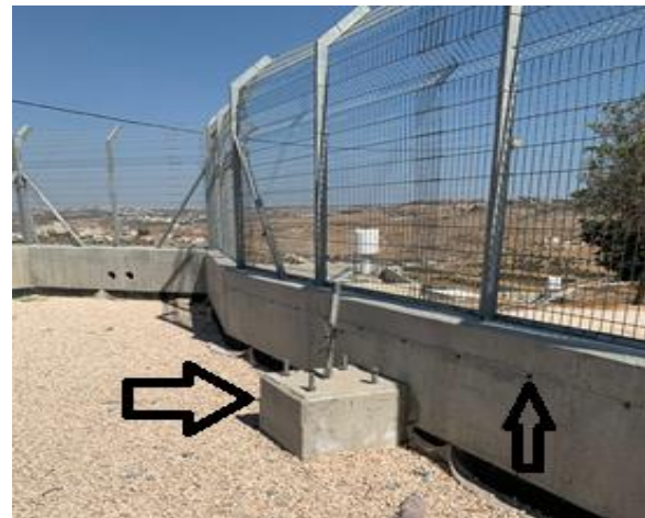
Tie rods locations must be filled. Electrical poles are not fixed
