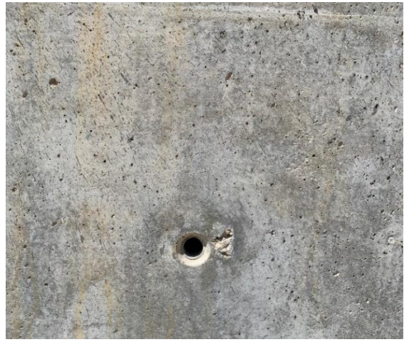
Tie rod holes must be repaired and filled
