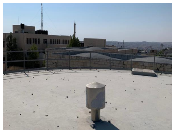
Air Vent are installed
