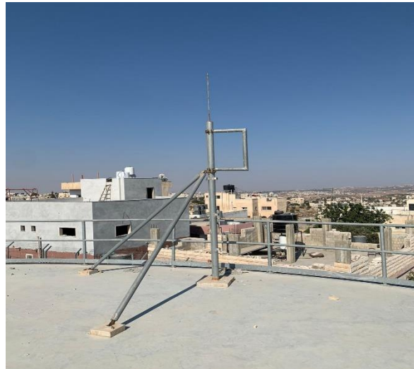
lightening is installed.
