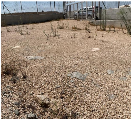
Reservoir yard level is not reached. Additional layers are required
