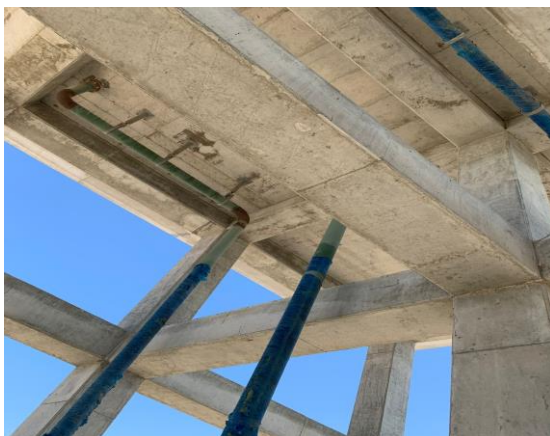
Tank during the filling- 50% filled. No Water leakage through floors, walls, or wall-floor joints.
