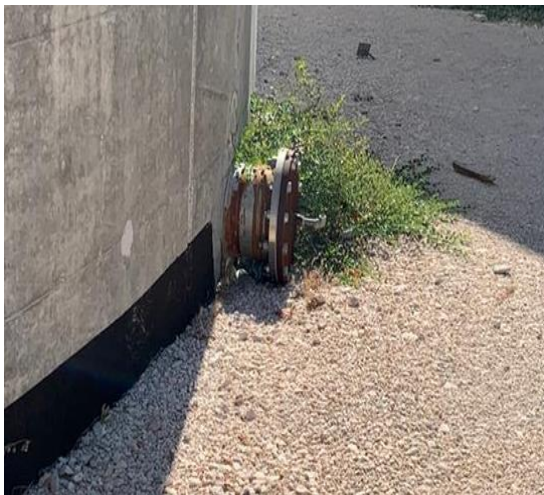
Rusted flanges have to be treated and insulated
