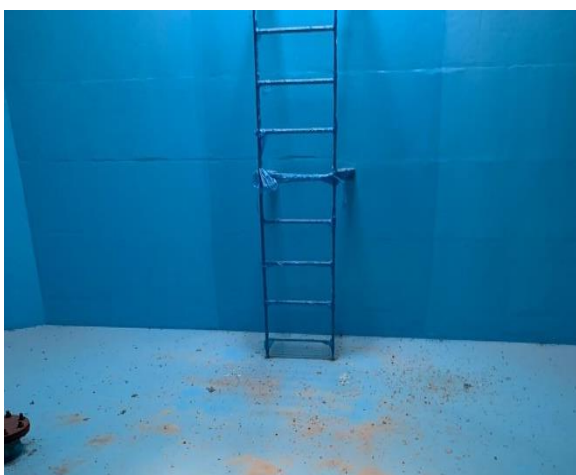
Tank is Epoxy coated from inside but need to improve its tightness
