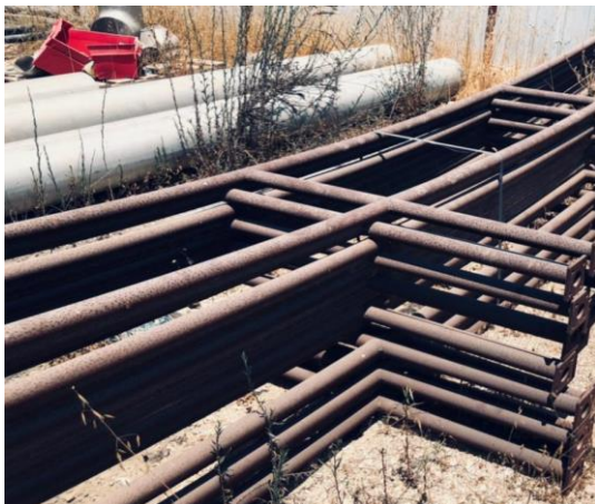
Handrails for Reservoir in bad condition but can be used
