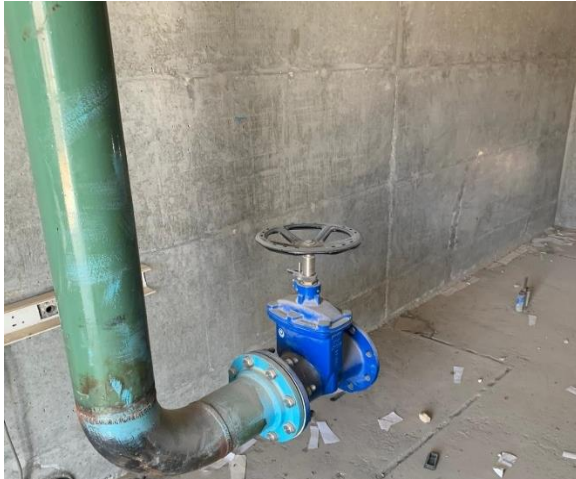
Inlet and Outlet Pipes must be treated from rust and insulated.
