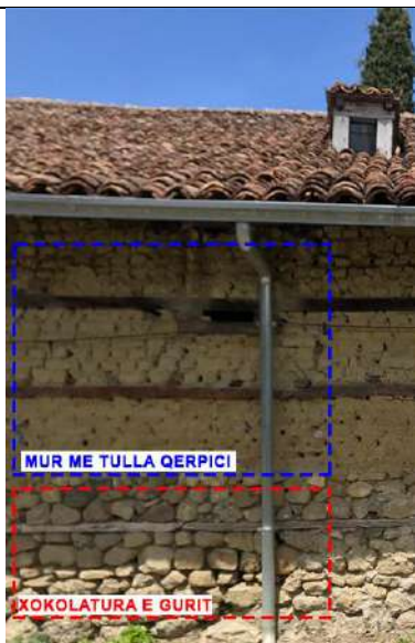
Fig. 25: The adobe wall layers
