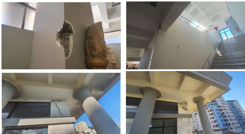
Fig. 22: Various deteriorations observed in the museum building, plaster cracks, damage to structural elements and plaster detachments.
