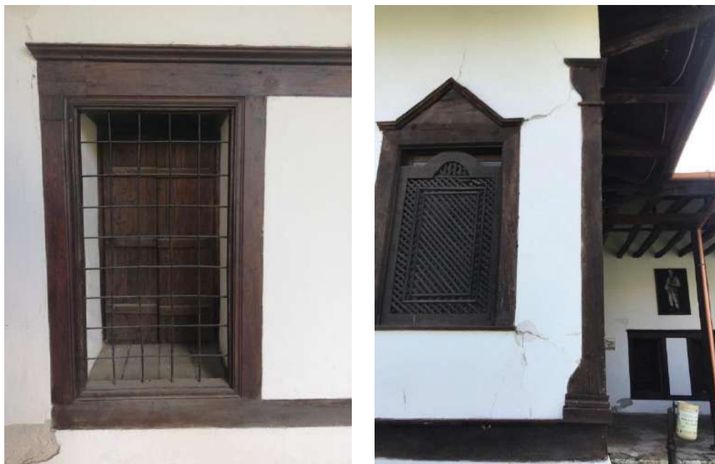
Fig. 18: Damaged wooden decorative elements
