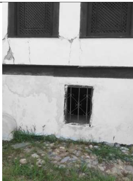
Fig. 26: The humidity of the building coming from the damaged drainage
