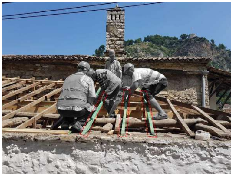
Fig. 24: Example of the replacing works for the damaged roof elements
