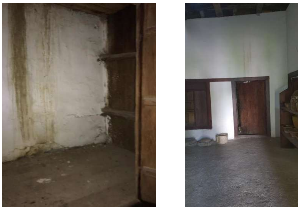
Fig. 19: Presence of moisture in the masonry
