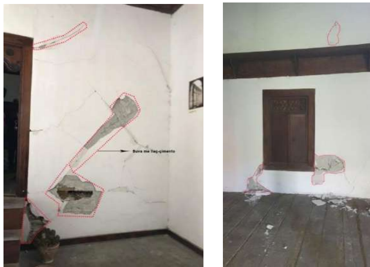
Fig. 27: Damage to the current plaster of the building
