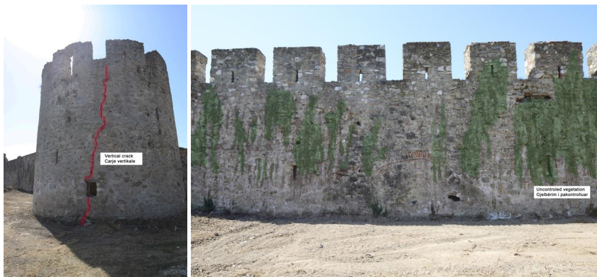
Fig. 30: Different deteriorations on the walls of the Bashtova Castle
