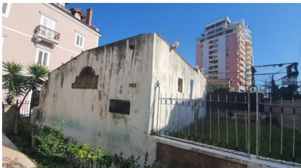
Figure 33. Presence of moisture and mold as well as deterioration of plaster on the facade
