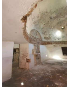
Figure 7 Detachment and drop of plaster
