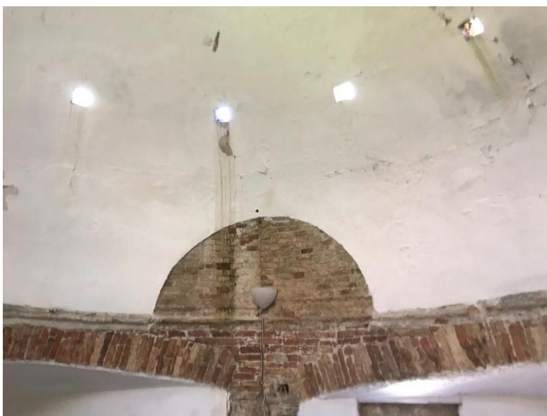
Figure 25. Stone masonry combined with brick in the waiting room of the hammam, the current condition
