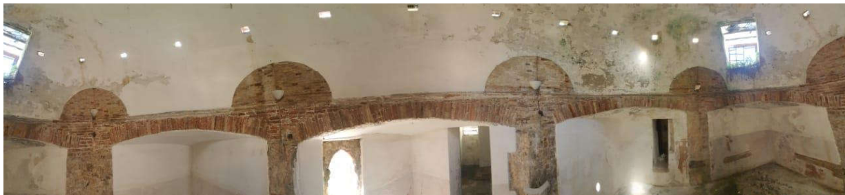
Figure 5 Presence of moisture, mold and vegetation
