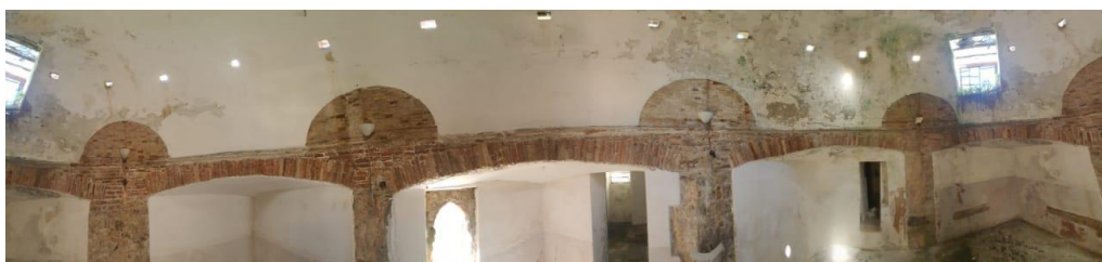
Figure 31. Presence of moisture, mold and vegetation
