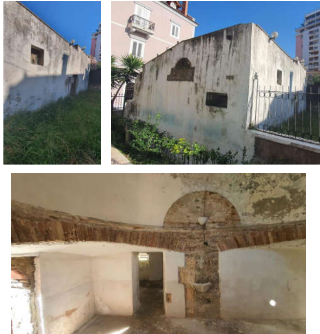
Figure 4 Stone masonry combined with brick, we encounter both in the premises inside and outside the Hammam.
