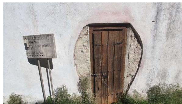
Figure 6 Degradation of the front door
