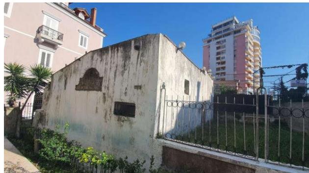
Figure 8 Presence of moisture and mold as well as degradation of plaster on the facade
