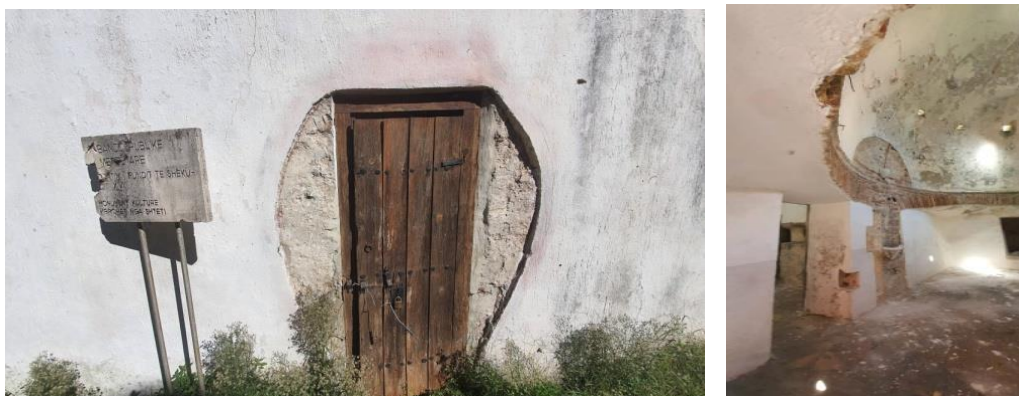
Figure 32. Entrance door deterioration; Detachment and drop of plaster
