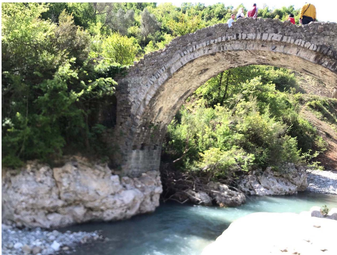
Fig. 11. Photo of the bridge, visible elements: the vault, the right niche, the parapet and the frontal retaining wall.
