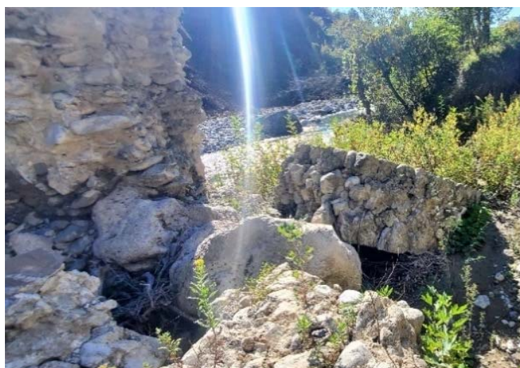
Fig. 16. Detached stone wall on the right side of the Kurcay bridge
