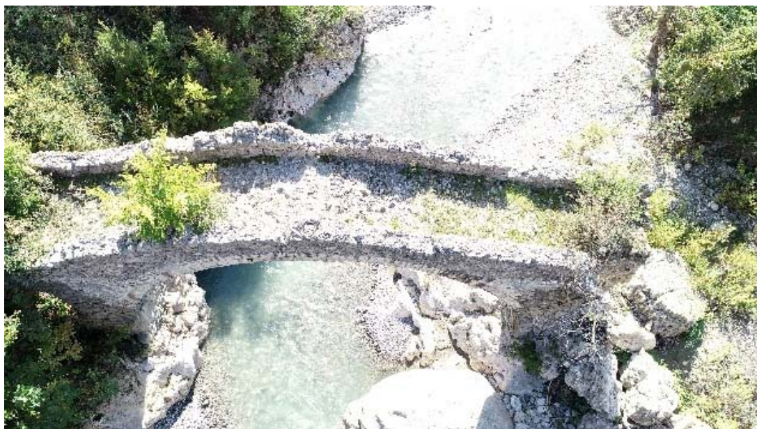
Fig. 21. Vegetation on the bridge and damaged parapet
