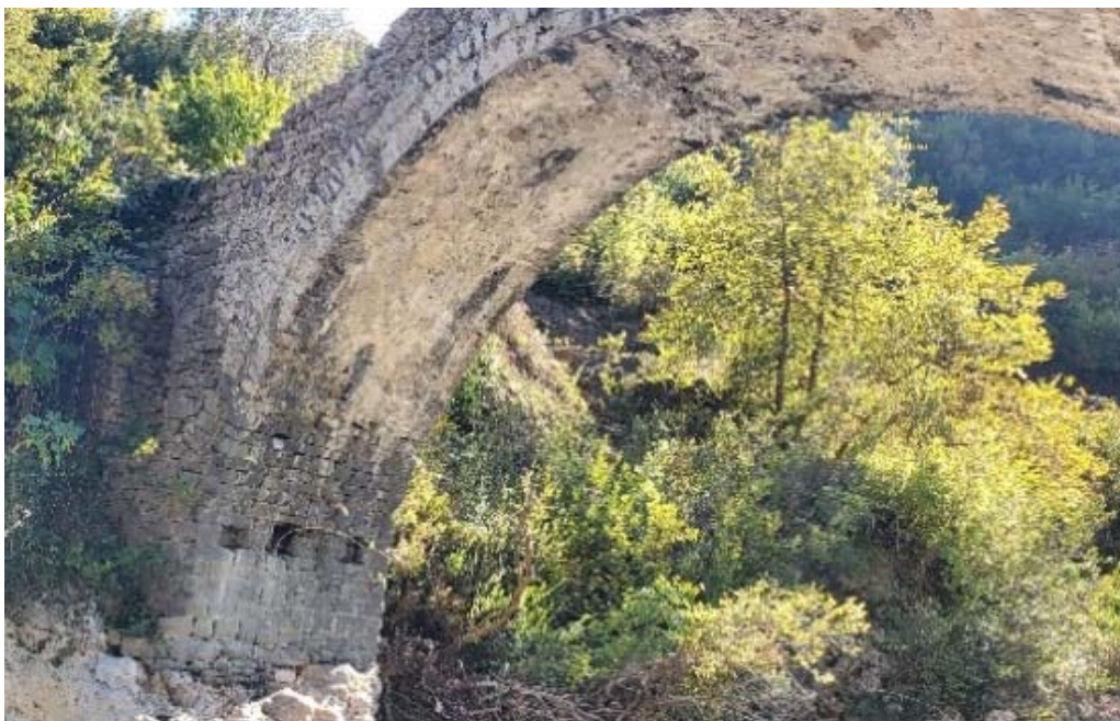
Fig. 27. Calcification and leakage of the mortar layer
