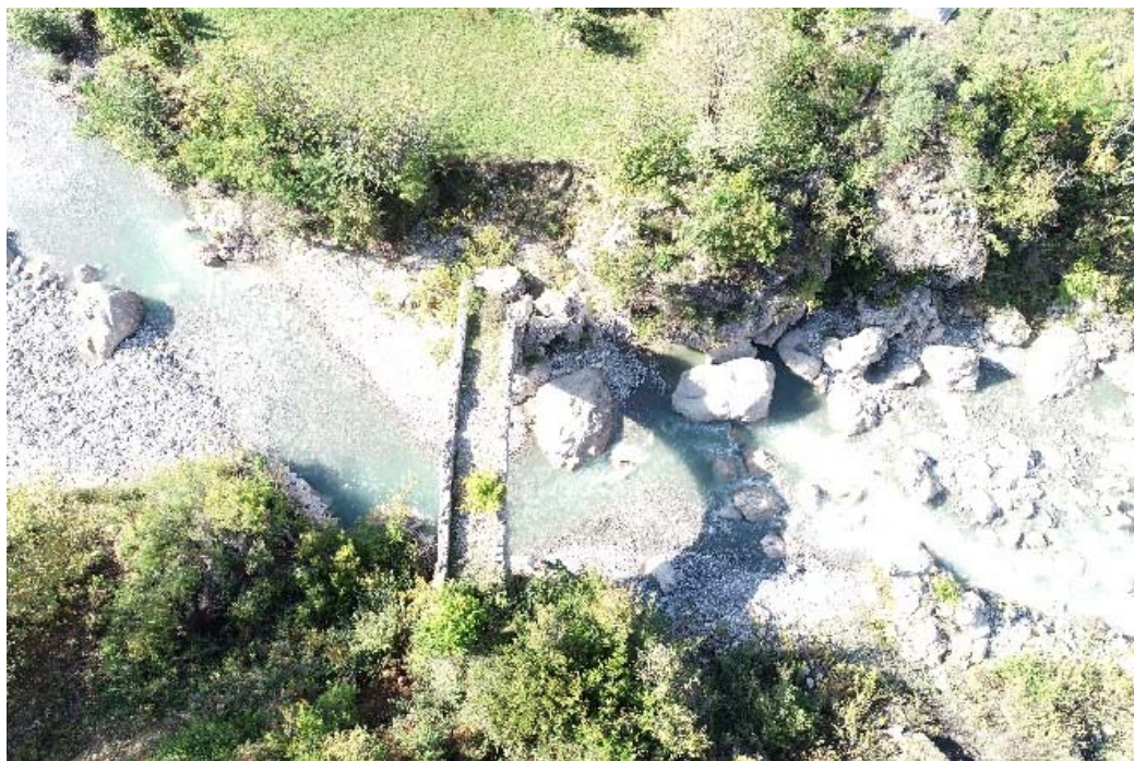
Fig. 18. Detachment of the Kurcaj bridge from the ground in the northern part
