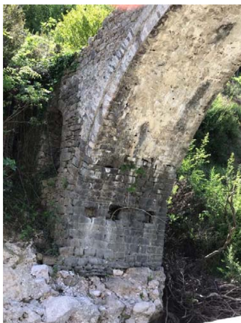
Fig. 14. Photos of the bridge, current condition: damages on the bridge's wings; stone wall decay; moss and humidity; deterioration of the vault stones due to reaction between atmospheric agents+humidity+river bank activity; inappropriate added layers (lime mortar) in an attempt to preserve the bridge.
