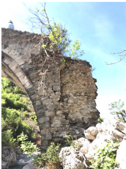
Fig. 26. Detached right wing of the bridge
