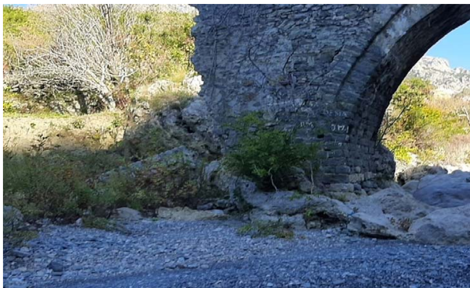
Figure 3: Cracking at an angle of 70 ° at the foot of the bridge from the side of the village Zgerdhesh, width > 10mm, filled with mortar.
