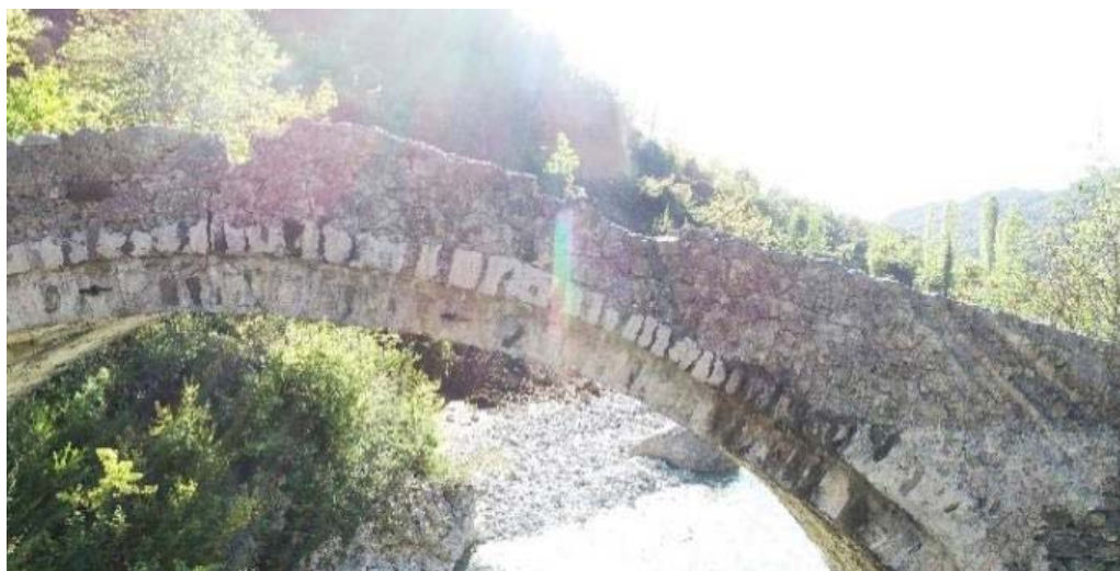
Fig. 28. Cracks on the vault
