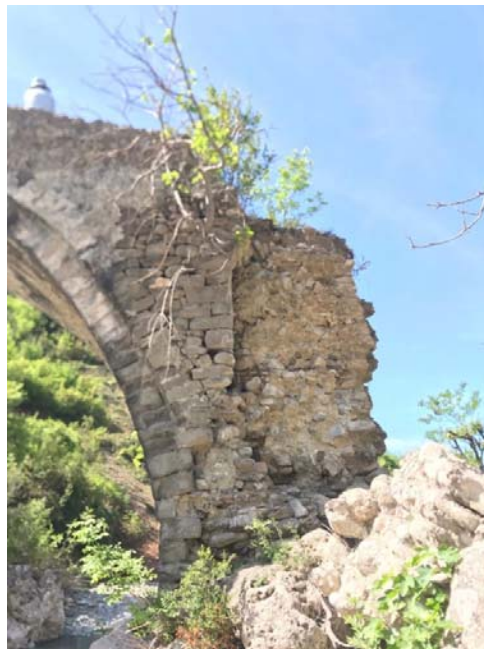
Fig. 14. Photos of the bridge, current condition: damages on the bridge's wings; stone wall decay; moss and humidity; deterioration of the vault stones due to reaction between atmospheric agents+humidity+river bank activity; inappropriate added layers (lime mortar) in an attempt to preserve the bridge.
