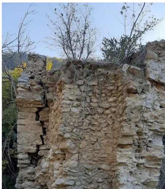
Figure 4 : Detachment of outer shell and inner fill material at the bridge abutment
