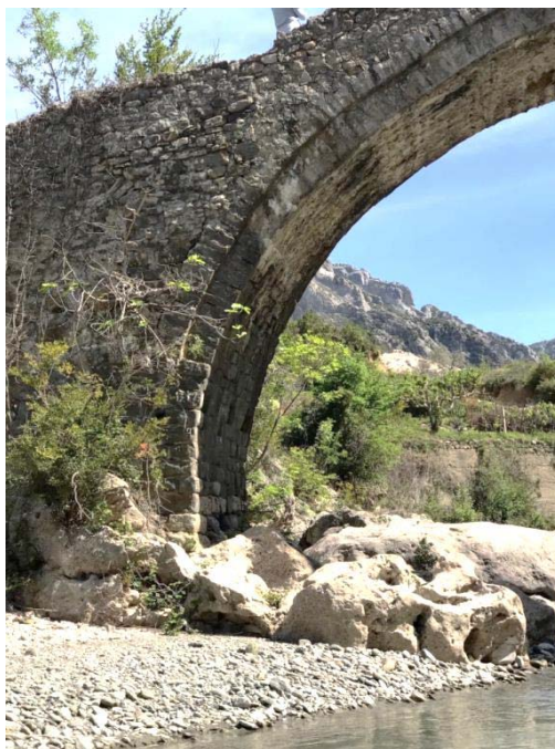
Fig. 25. The left arm of the bridge rests on the stone foundations
