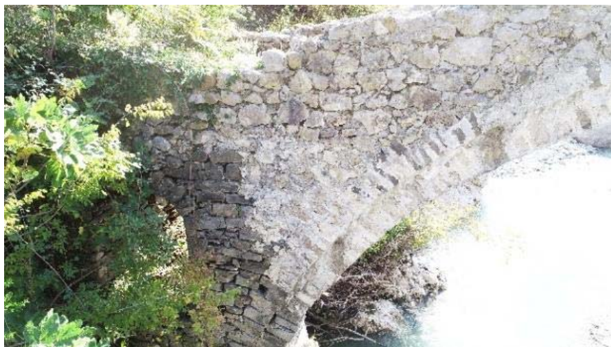
Fig. 29. Repairs during different periods of time adding inappropriate layers, which, by interacting with chemical and atmospheric agents have damaged the foundations of the Kurcay bridge
