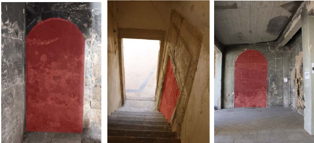
Fig. 4-1 The three filled openings
