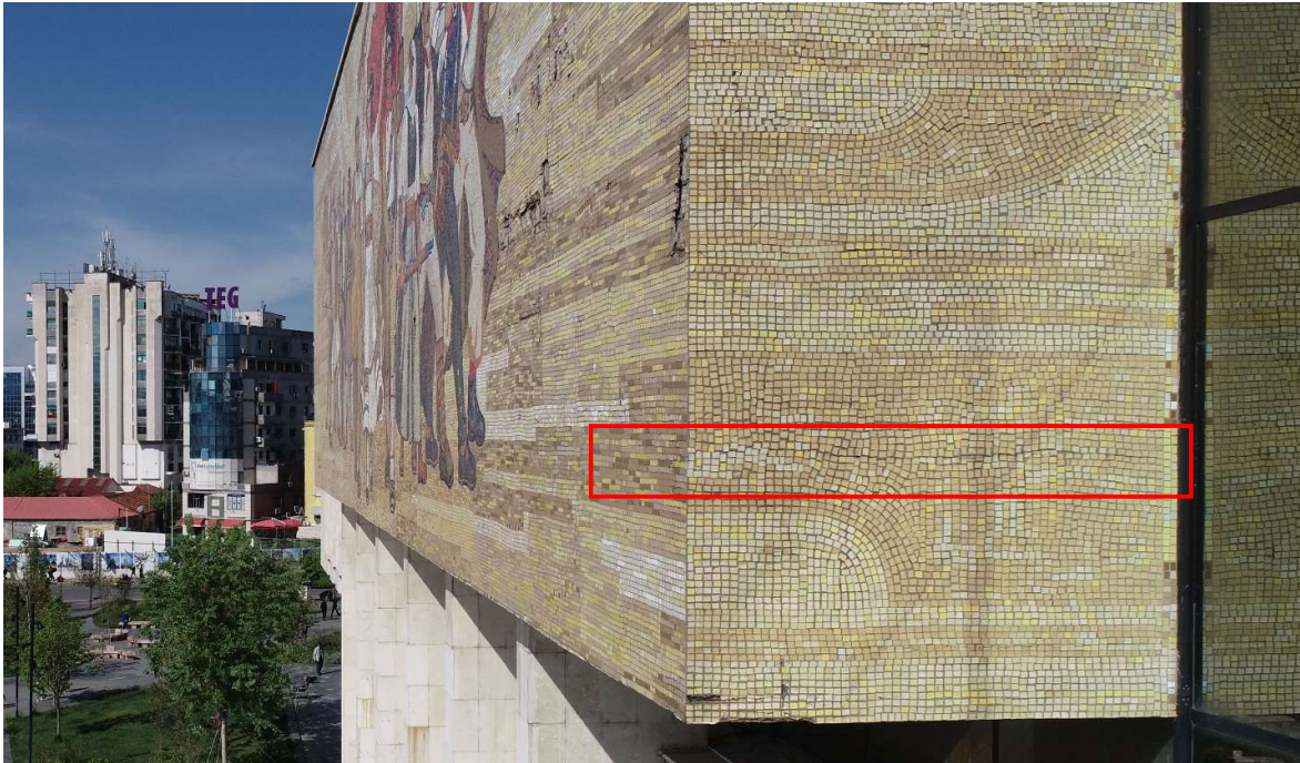
Fig. 26 – Cracks presence
