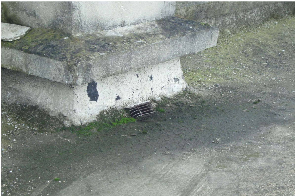
Fig. 36 – Drain images that are not according the standard and totally amortized
