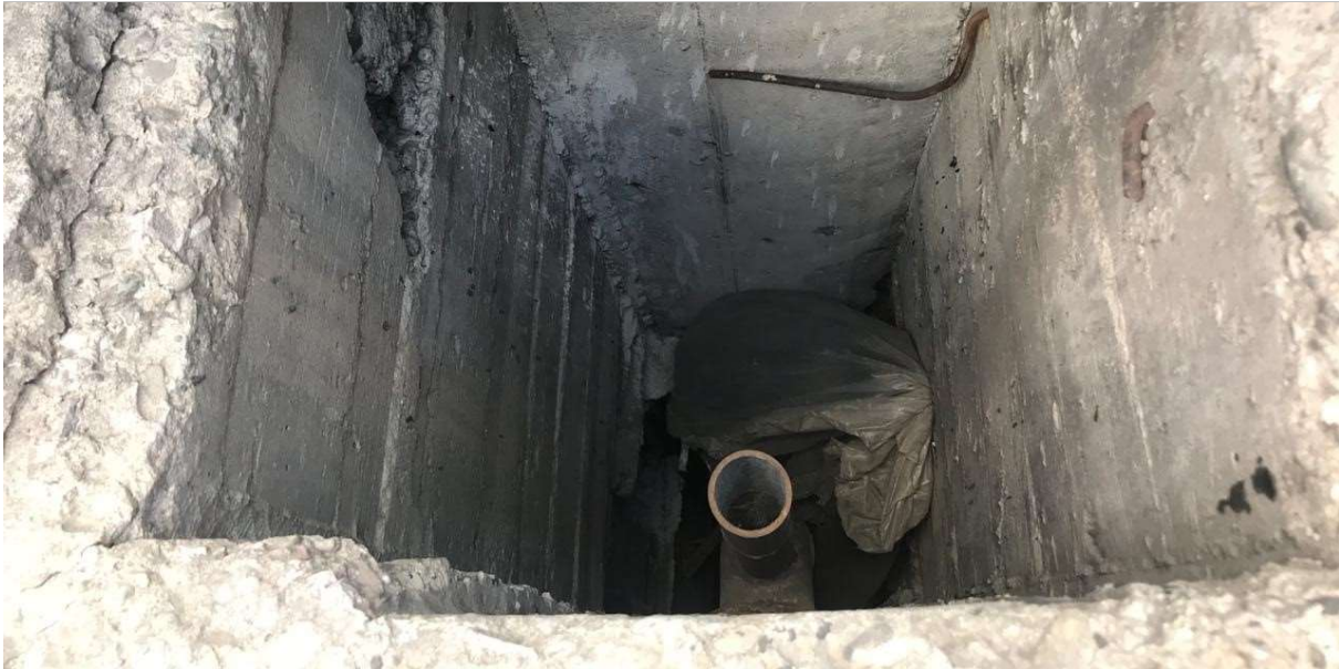
Fig.37- the pit picture of the rainwater discharge columns which is in a position and dimension inaccessible for inspection. It is distinguished the inadequate technique of building of the pit as well as the degradation of the cast iron pipes, their joint etc.
