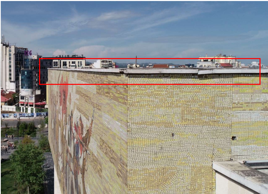
Fig. 25 – Deterioration of the roof parapet (handrail)
