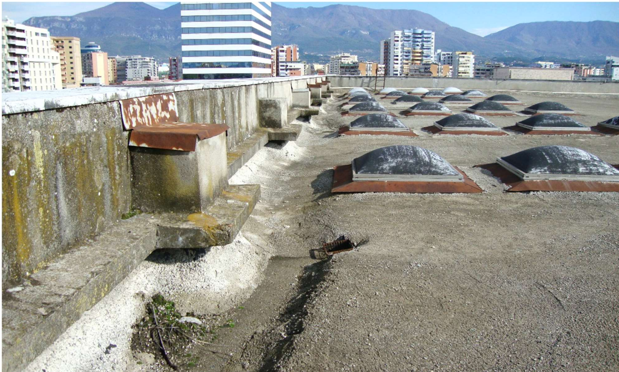
Fig. 35 – Drain images that are not according the standard and totally amortized
