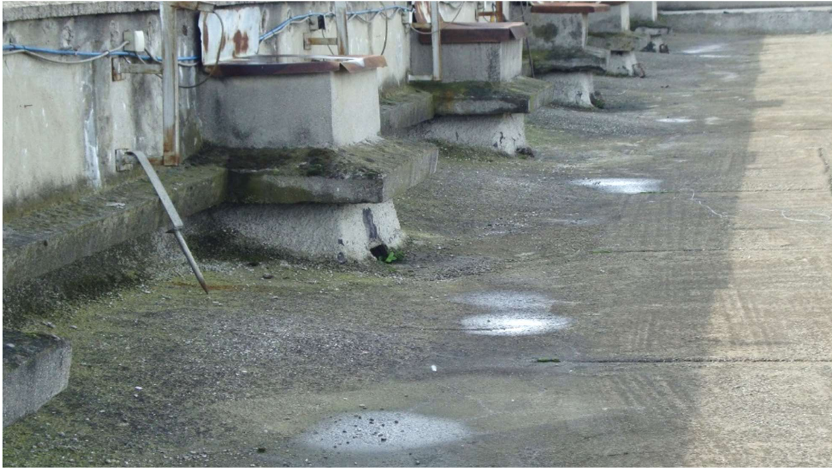
Fig. 34 – Drain images that are not according the standard and totally amortized
