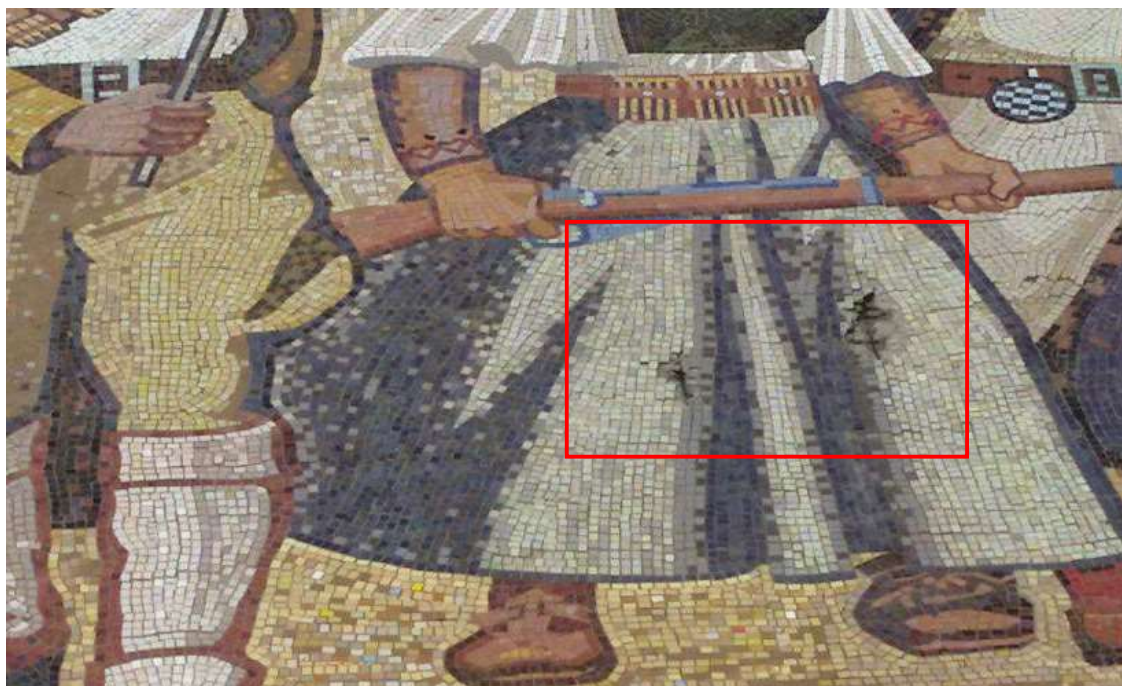
Fig. 28– Exposed metallic grill
