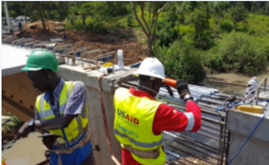
Independent QA inspection of welded splice
