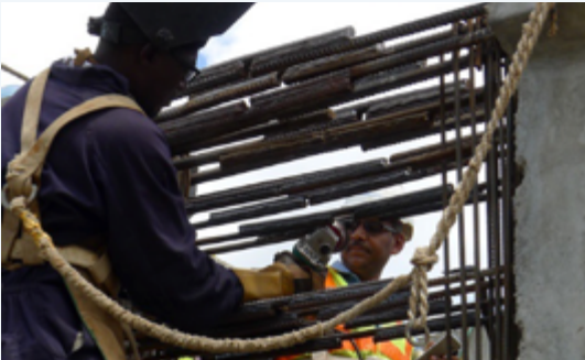
Visual in situ welding inspection
